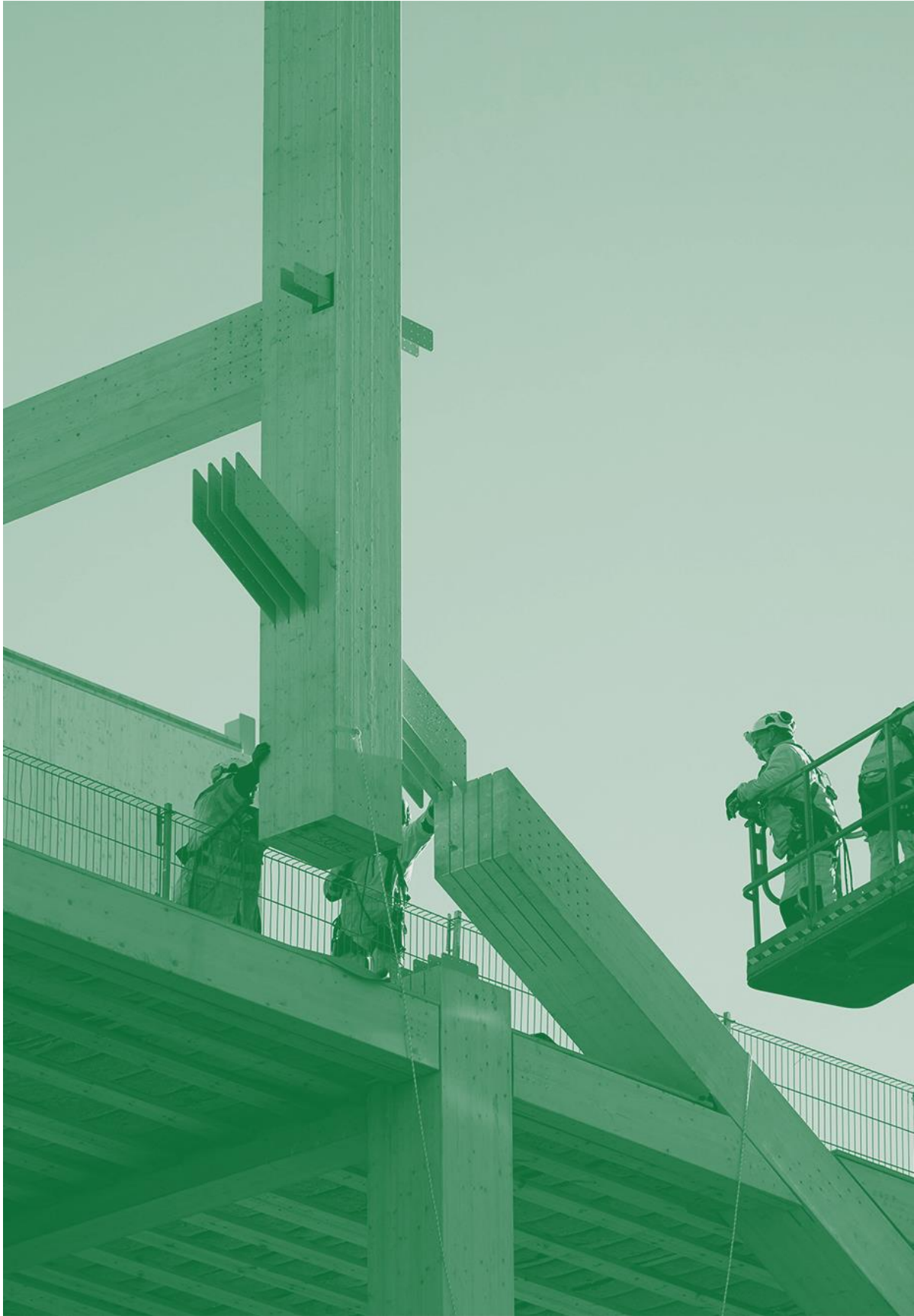
Figure 13: IKEA-like assembly of a highrise building, Mjøstarnet. Photo: Jens Haugen.
